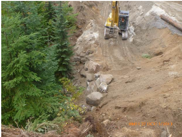
Photo 1. Armoring of the culvert outlet at Stn. 2056.0 – Oct 1, 2013
