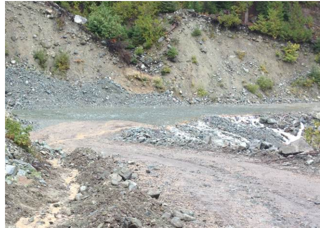
Photo 2. Conditions at Truckwash Creek on Sept 30 th . Minor input of sediment laden water did not result in WQ exceedence.
