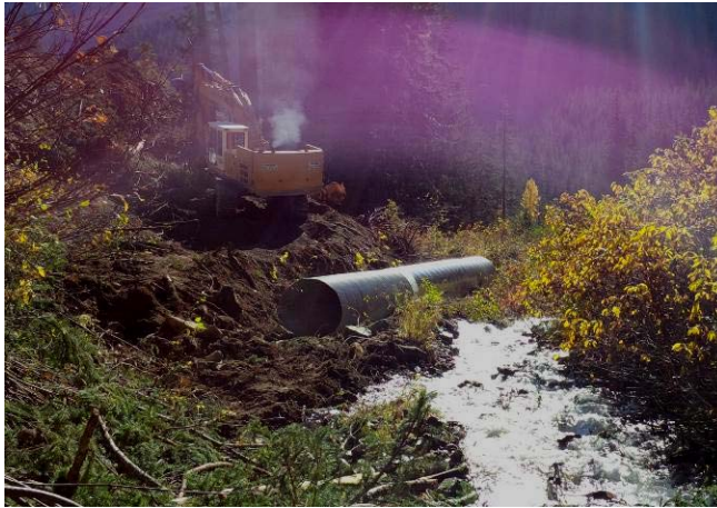
Photo 1. Culvert installation and cofferdam at Stn. 1+430 (Oct 16, 2013).
