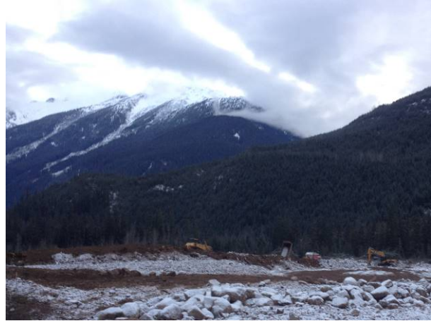
Photo 4. Construction of the visual/auditory berm at the future construction camp location. (Dec 11, 2013).
