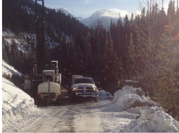
Photo 2. Borehole drilling on the access road north of the ULRHEF intake. (Dec 9, 2013).
