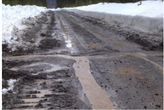
Photo 2. Conditions of the FSR following the installation of shallow ditching and water bars to control surface runoff and direct water to vegetated areas for infiltration. (April 5th, 2013).
