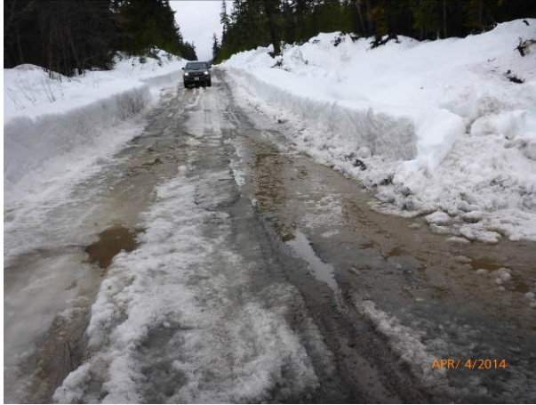
Photo 1. Overview of the results of snow blowing and surface runoff and ponding concerns. Notice there are no snow berms resulting from snow removal works. (April 4, 2013).
