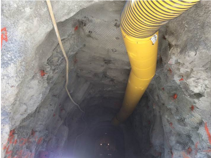
Photo 1. Tunneling works at the tunnel portal entrance. (July 9, 2014).
