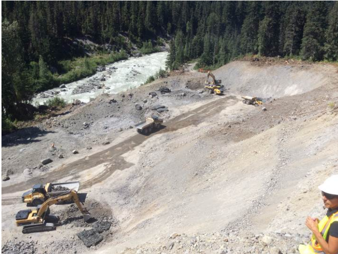
Photo 3. Excavation of the ULRHEF powerhouse footprint (July 9, 2014).
