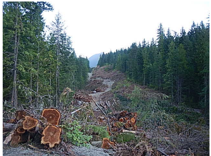
Photo 6. Clearing and access track construction in Segment 7 (July 11, 2014).
