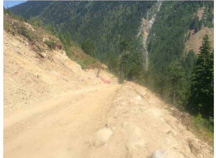
Photo 2. Construction of the BDR intake access road. (July 11, 2014).
