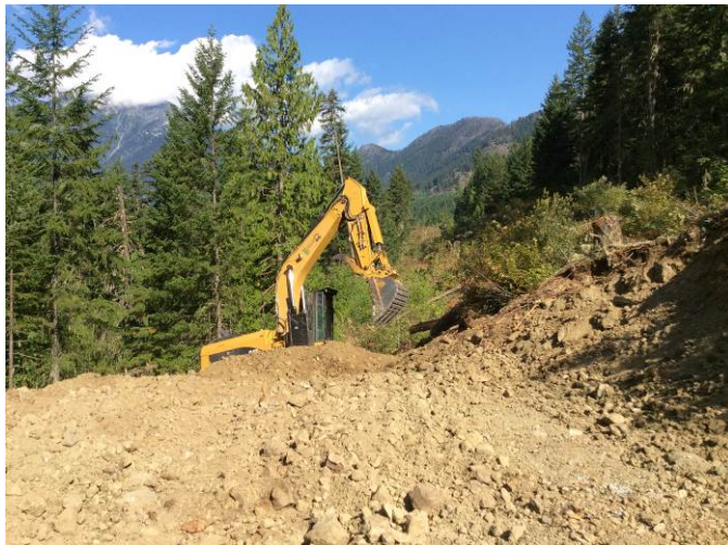
Photo 5. Road construction in Segment 7 (July 22, 2014).
