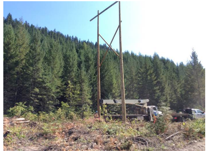
Photo 6. Poles installation in Segment 4 (July 19, 2014).
