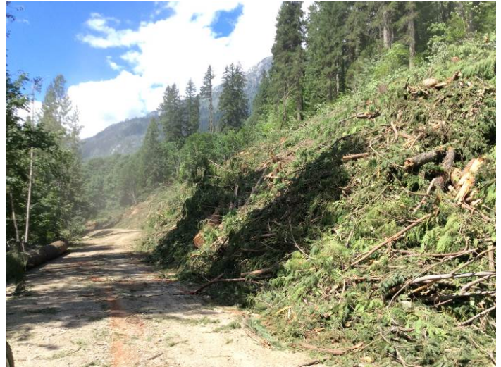
Photo 6. Results of hand clearing in Segment 5 (August 6, 2014).
