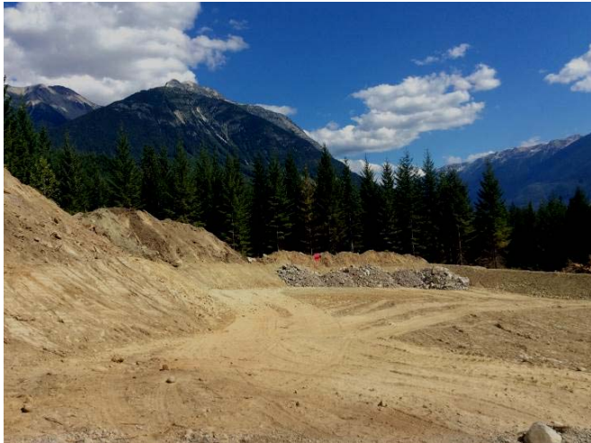
Photo 1. Preparing BDR-4 as a temporary storage area for PAG generated from the Boulder Intake access road construction. This area will be used once works resume following the removal of the Stop Work Order (August 6, 2014).
